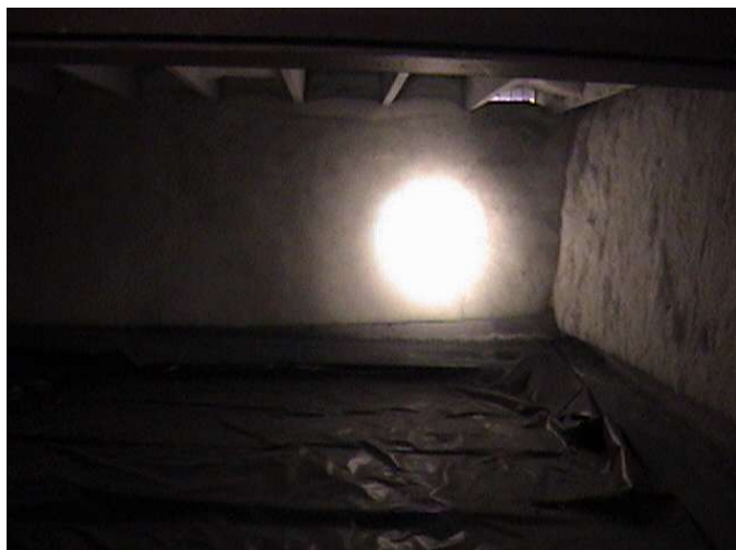
Crawl space appears to be well insulated and ventilated.
