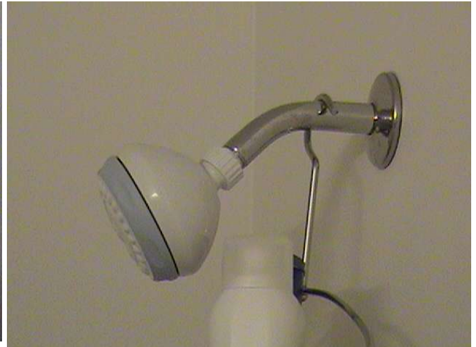
Repair: The shower head plumbing in the main bath is loose.
