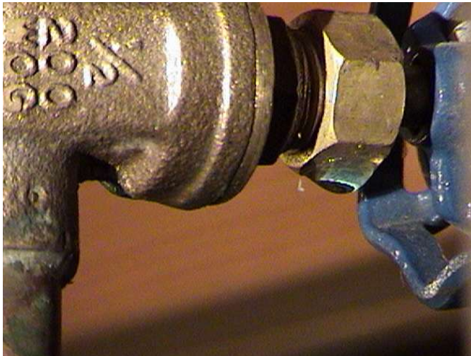
Also the valve in the copper line going to the out side on the west side of the home is leaking. This is in the crawl space.
